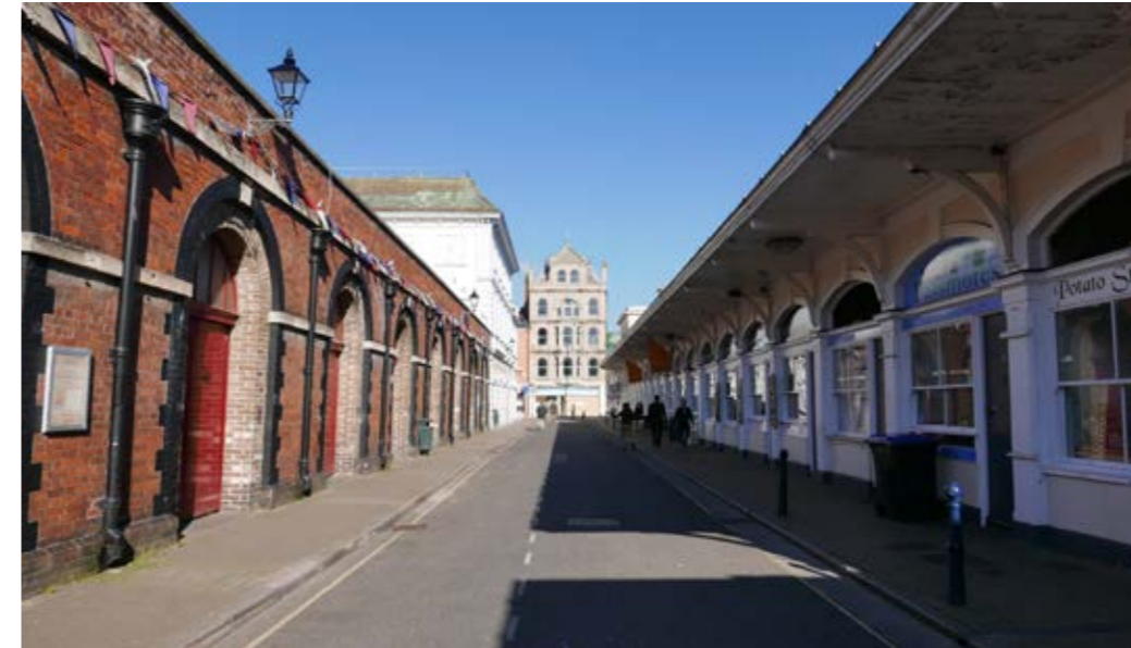
Image 4: Existing external View of the Pannier Market & Butchers Row
