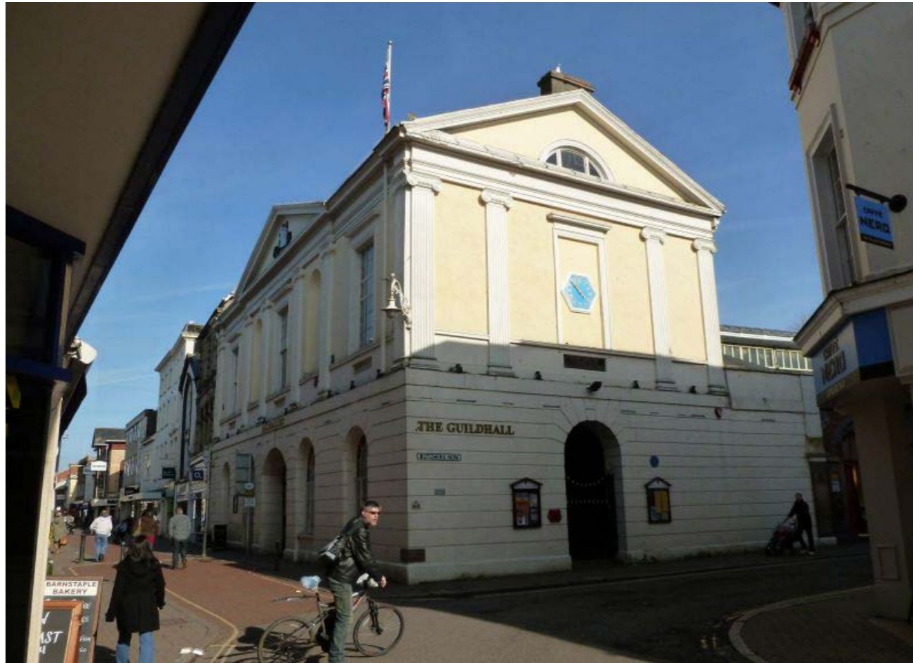
Image 15: View of the Guildhall along High Street
